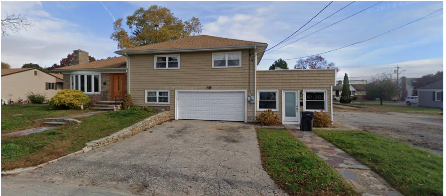
STREET VIEW (Kearney Street)
